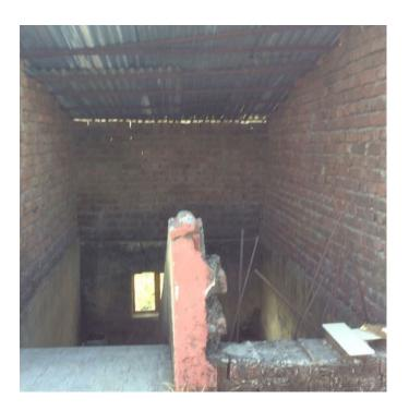
The staircase needed a roof. During the monsoons, rain water would cause great discomfort. Work is underway to put a roof over the staircase.
