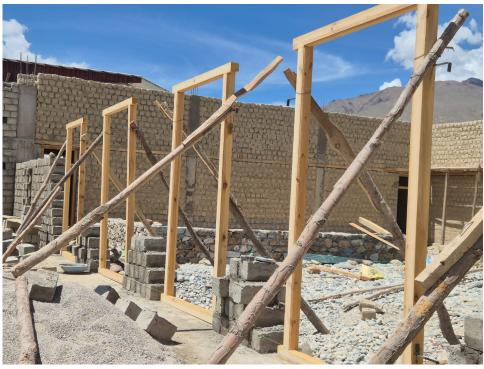
The installation of interior window and door frames has been initiated as per the approved architectural layout. Frames are aligned vertically and horizontally using water levels and plumb lines to ensure accuracy in placement. Proper anchoring methods are employed to secure the frames firmly within the wall cavities, thereby maintaining structural stability and alignment.
