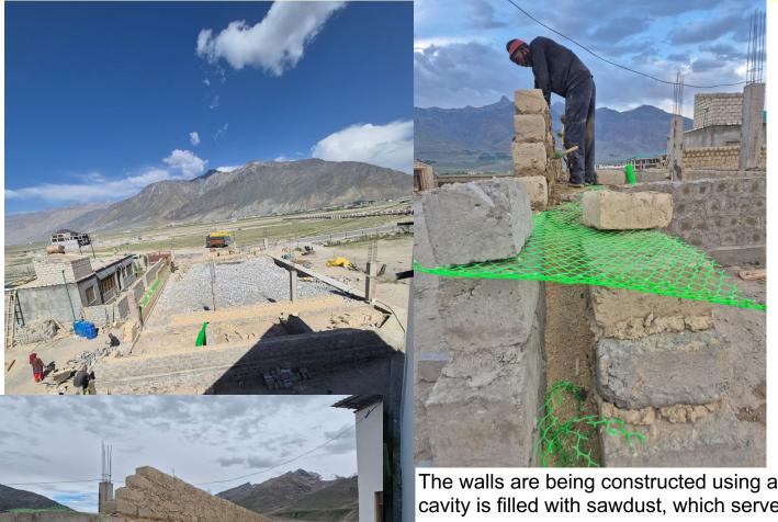
The walls are being constructed using a cavity-wall system. The cavity is filled with sawdust, which serves as an insulation material. The sawdust is compacted (rammed) in layers to achieve the required density and stability, resulting in a total wall thickness of 24 inches. To enhance structural integrity, geo-mesh reinforcement is installed at every 4 feet of height, effectively tying the two wall leaves together and ensuring overall strength and durability of the wall system.
