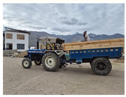
Exterior window frames, fabricated at the local workshop as per approved design specifications, have been transported to the construction site. Care was taken during handling and transportation to prevent damage, bending, or warping of the frames. The frames will undergo inspection upon arrival to verify dimensional accuracy, surface finish, and structural stability prior to installation. This step ensures quality compliance and readiness for integration into the building envelope.
