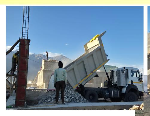
After raising the foundation up to 3 feet above ground level, we have started filling the foundation with gravel of random sizes. The filling is carried out with proper levelling using shovels, and labourers have ensured an even surface.
