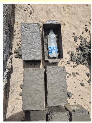
Workers carefully prepare thermal bricks by filling empty plastic bottles with salt and subsequently adding water to enhance their thermal mass. These filled bottles are then cast into concrete blocks, forming composite thermal bricks.
